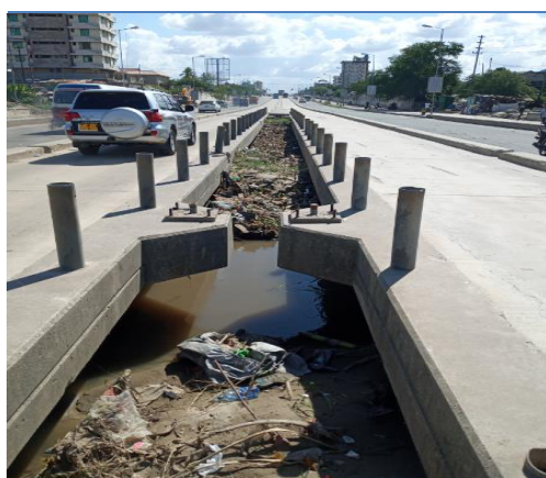
Figure 3.4 A: Shows Part of the Observed Jammed Condition at Jangwani Bridge. Photo taken on 13 th July, 2020
